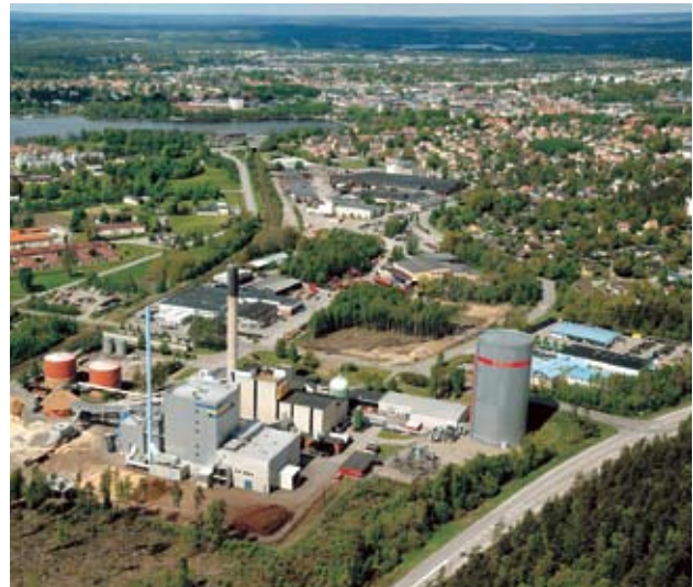
View over the CHP plant, with Växjö in the background.
